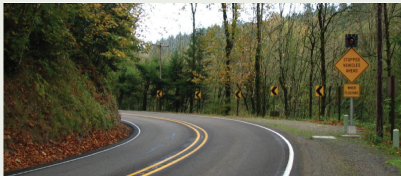
Clear delineation of curves is another low-cost safety improvement.
